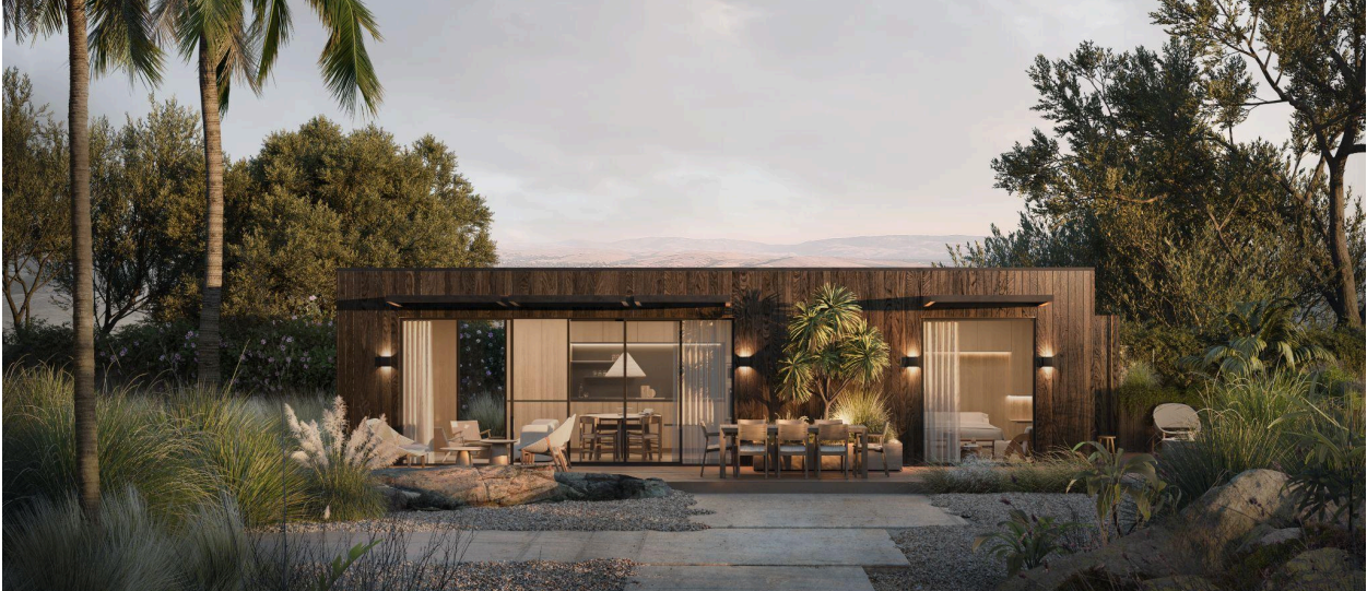
Exterior view of ikkon 1 - 432 sqft 1Bed 1Bath ADU - 1 of 3 available models for a short term solution
